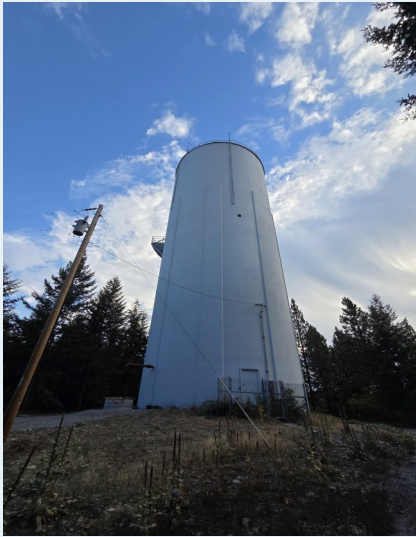
Bayview Water Tower, located in Farragut State Park
