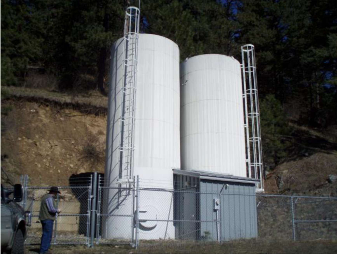
Figure 5. Cape Horn Estates Reservoir
