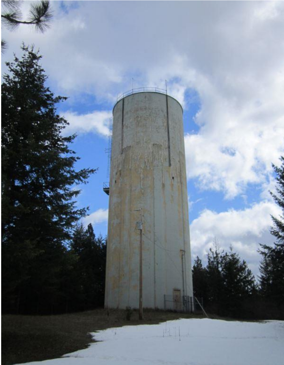
Figure 3. Farragut Reservoir Tank (225,000 gal)-July 2019
