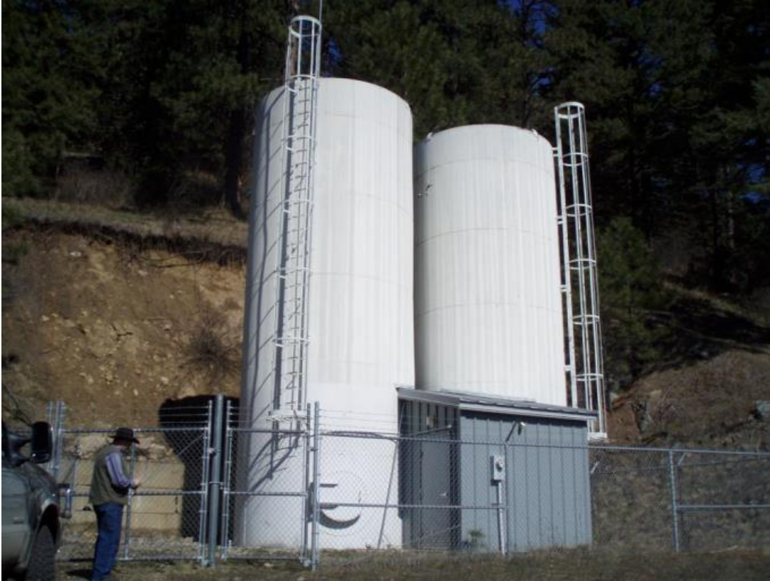
Figure 6. Cape Horn Estates Reservoir
