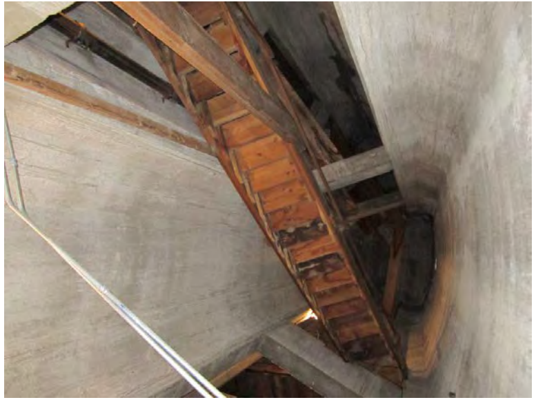
Photograph 24: Farragut Tank internal stairway access
