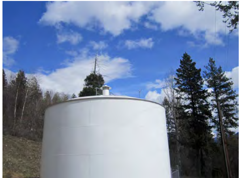
Photograph 56: Pend Oreille tank vent w screen
