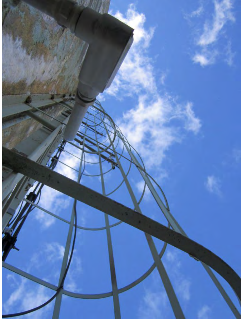
Photograph 34: Farragut Tank access ladder
