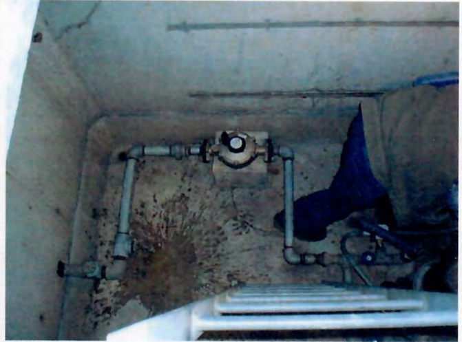
Photograph 2: Dromore Booster Vault
