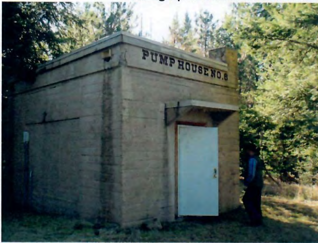
Photograph 5: Pump house for Well 8
