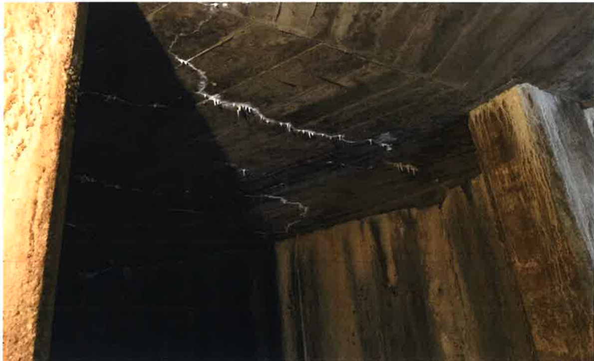
Figure 4 – Cracks with Small Stalactites Forming on the Bottom of the Tank Floor
