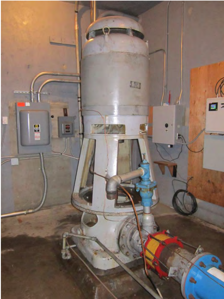
Photograph 3: Well 7 water lubed VTLS
