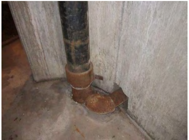
Photograph 26: Farragut Tank overflow
