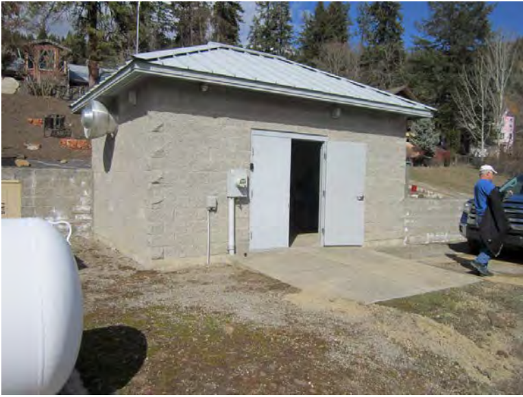
Photograph 65: Limekiln booster pump building
