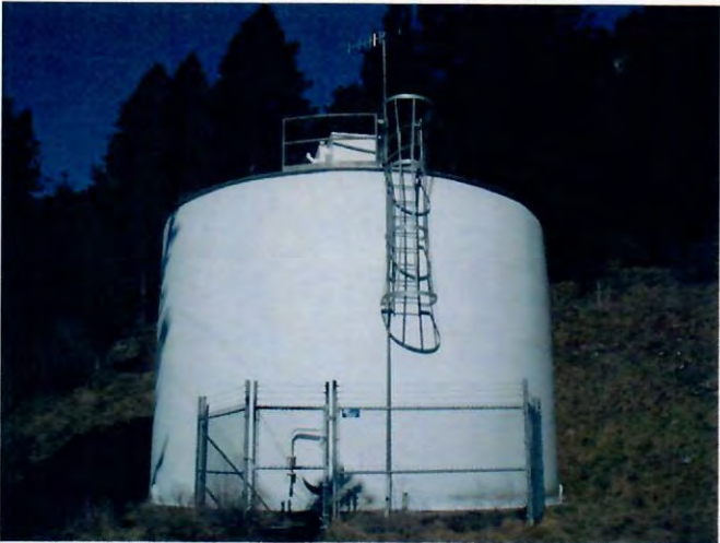
Photograph 15: Pend Orielle Pines Reservoir
