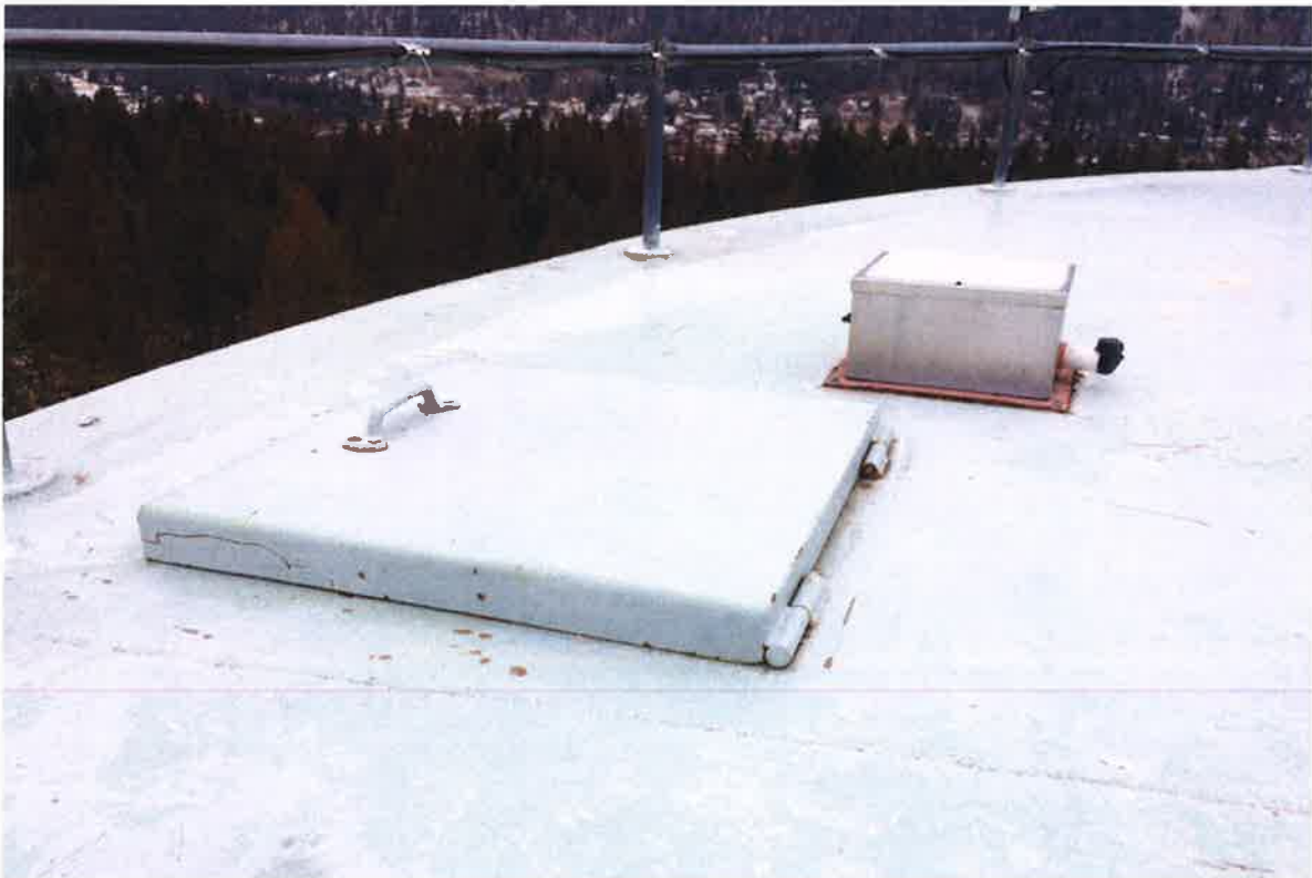
Figure 8 – Reservoir Roof and Access Hatch
