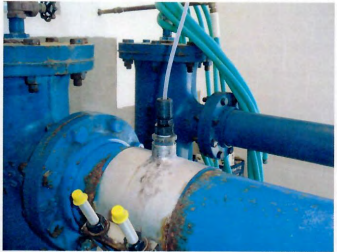
Photograph 12: Injection site for Cape Horn distribution
