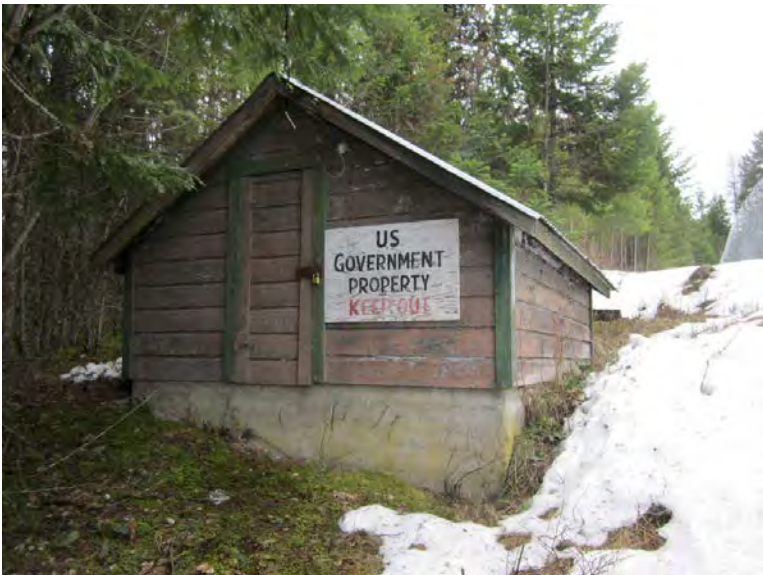
Photograph 51: Farragut tank PRV
