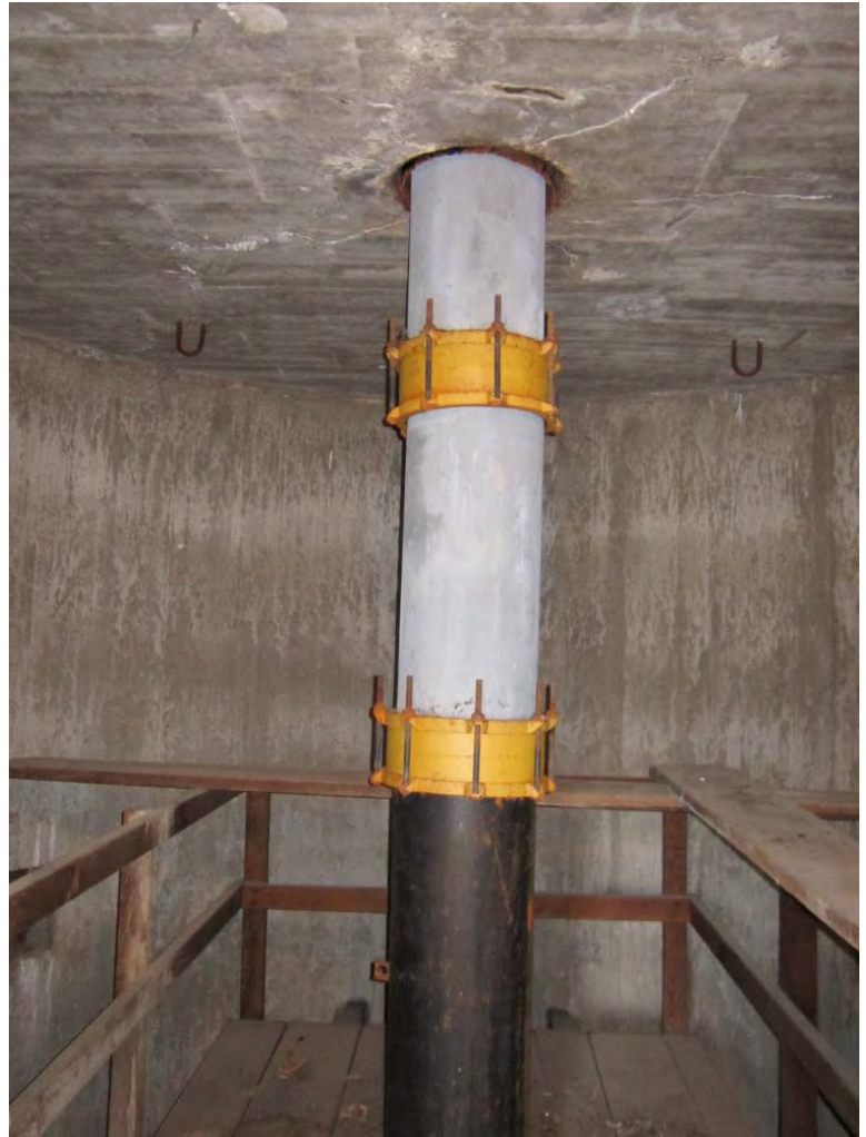
Photograph 32: Farragut Tank shared inflow/outflow to tank floor
