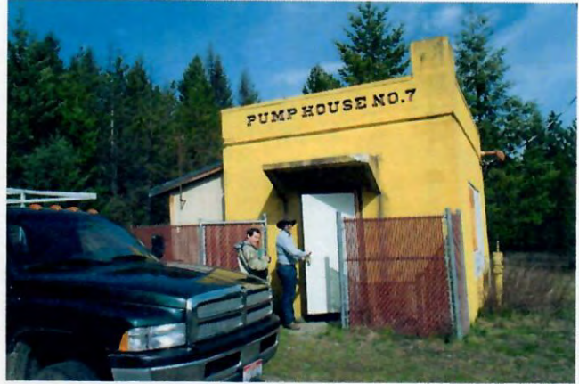
Photograph 20: Pump house for Well 7
