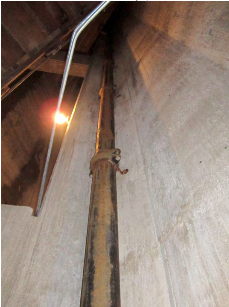
Photograph 27: Farragut Tank overflow
