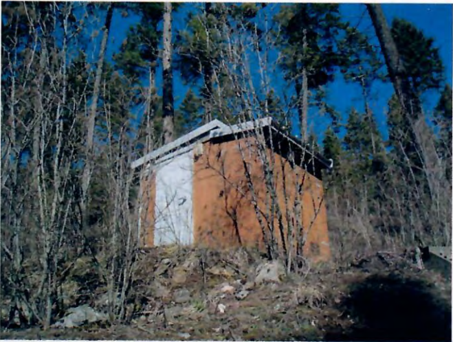
Photograph 16: Cape Horn Estates Booster station
