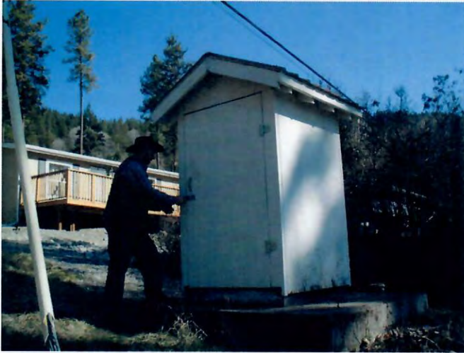
Photograph 1: Dromore Booster Station
