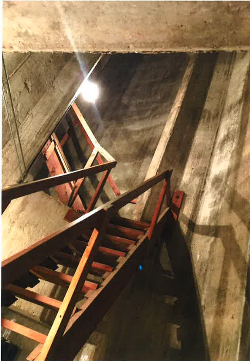
Figure 6 – Interior View of Access Stairs
