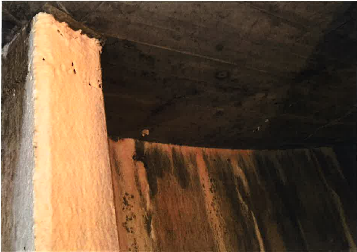
Figure 4 – Cracks with Small Stalactites Forming on the Bottom of the Tank Floor
