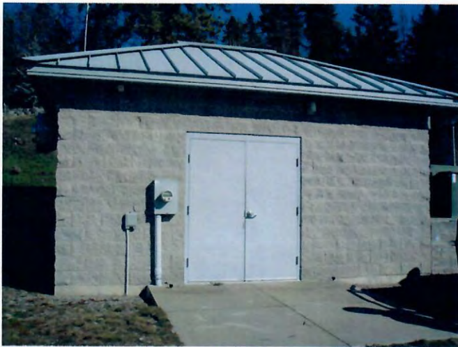
Photograph 7: Cape Horn Booster Station
