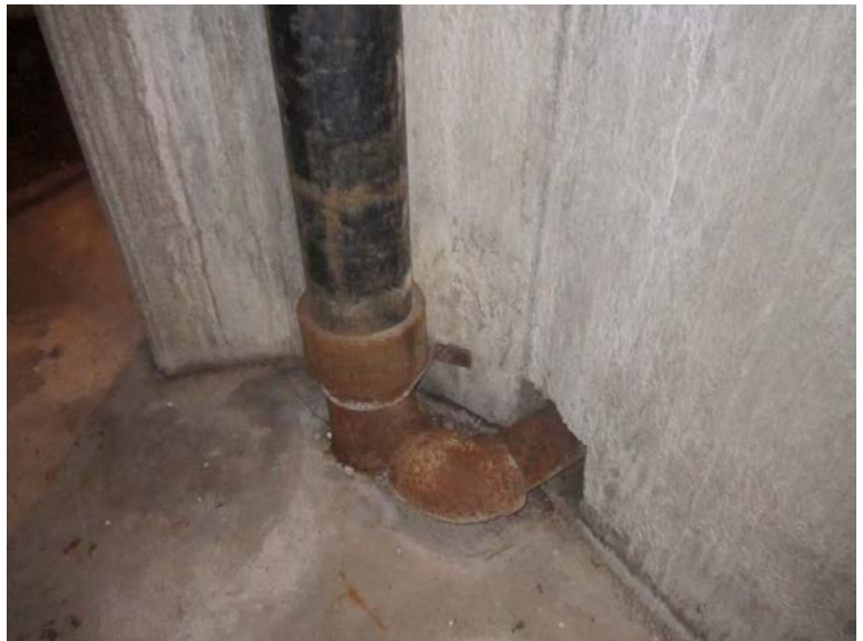
Photograph 26: Farragut Tank overflow
