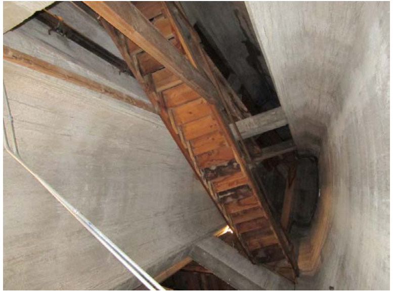
Photograph 24: Farragut Tank internal stairway access
