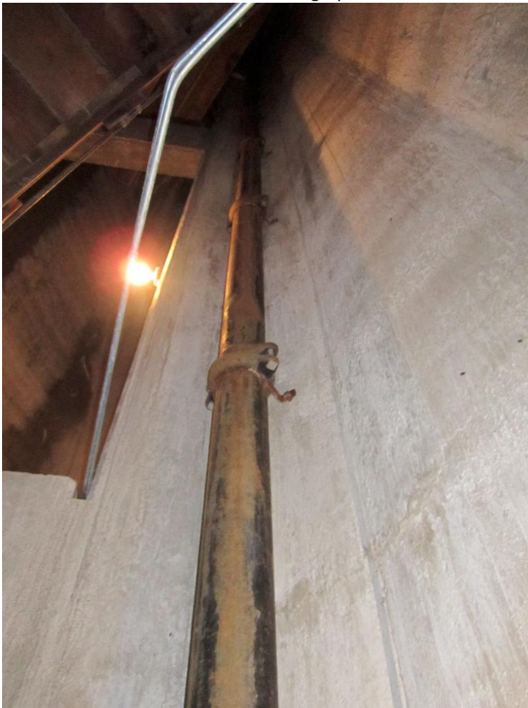
Photograph 27: Farragut Tank overflow
