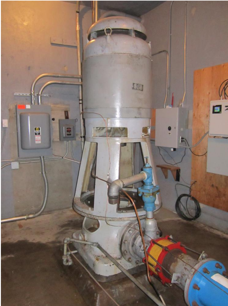
Photograph 3: Well 7 water lubed VTLS
