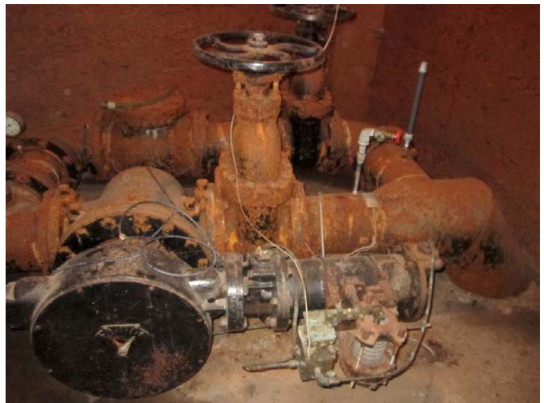
Photograph 30: Farragut Tank shared inflow/outflow isolation valves
