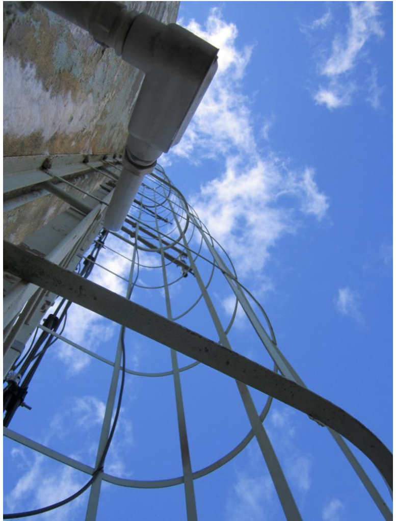
Photograph 34: Farragut Tank access ladder
