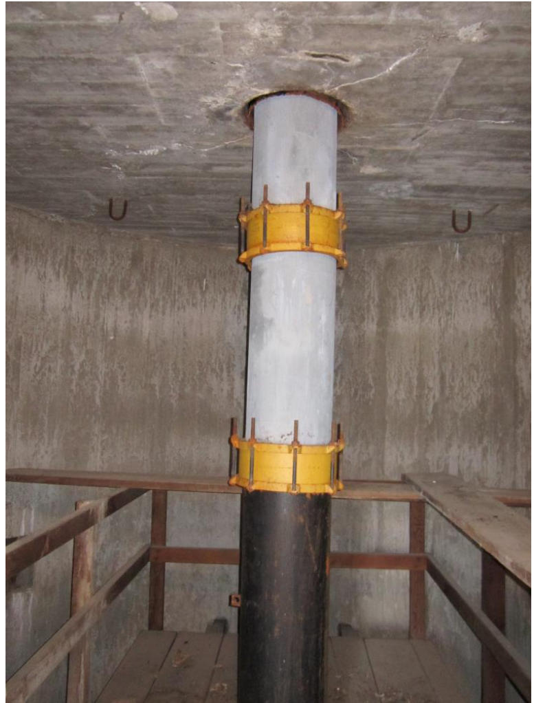
Photograph 32: Farragut Tank shared inflow/outflow to tank floor
