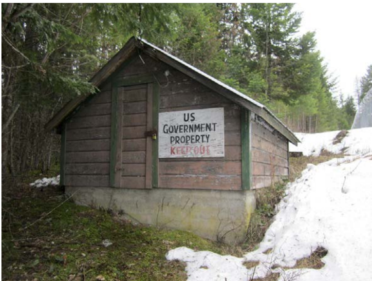
Photograph 51: Farragut tank PRV
