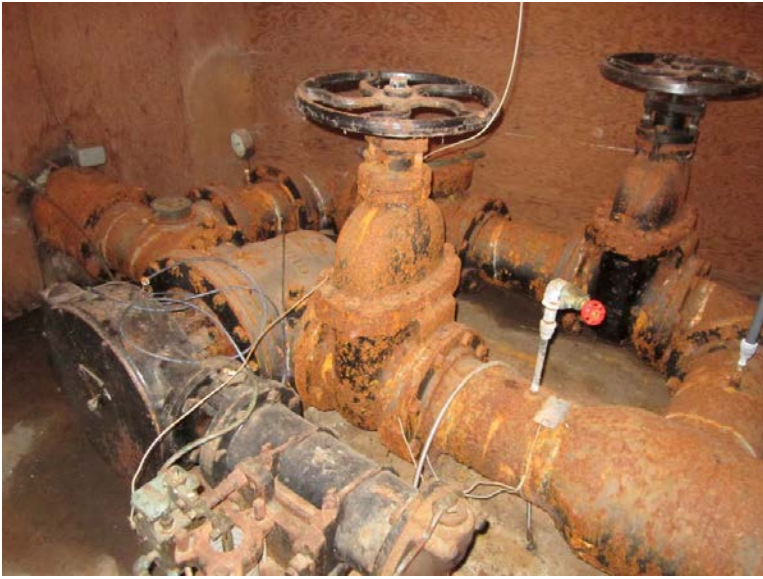
Photograph 31: Farragut Tank shared inflow/outflow isolation valves
