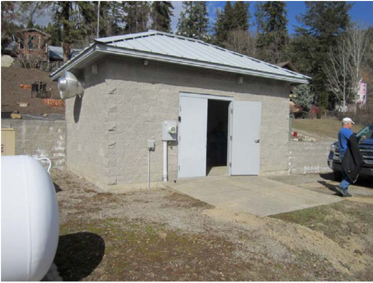
Photograph 65: Limekiln booster pump building
