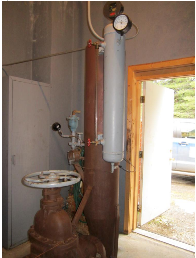
Photograph 8: Well 7 air/pressure relief (torpedo casing)
