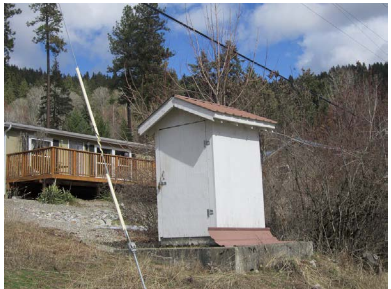
Photograph 52: Dromore booster station
